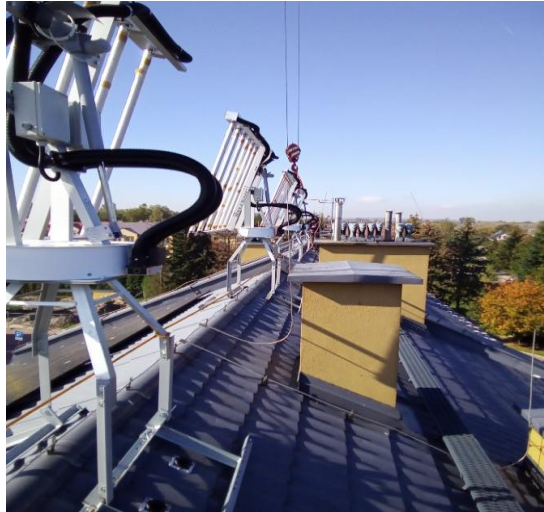
Sun-tracked solar collectors
