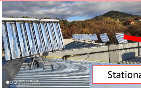
Solar collectors on trackers
