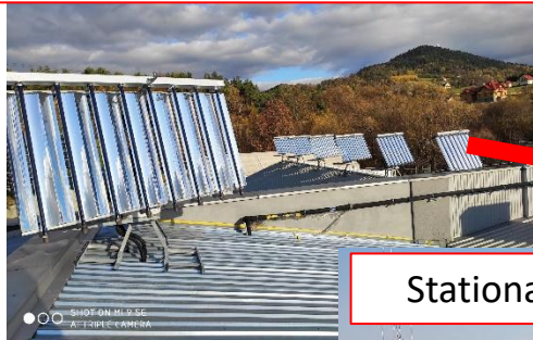
Solar collectors on trackers
