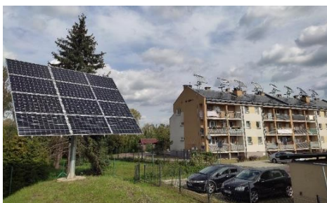
RESHeat system Installation in Cracow
