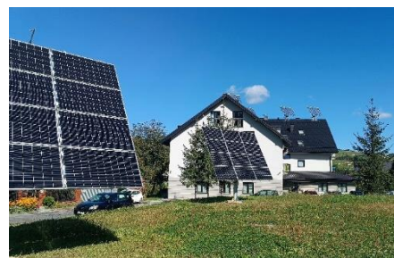
RESHeat system Installation in Limanowa
